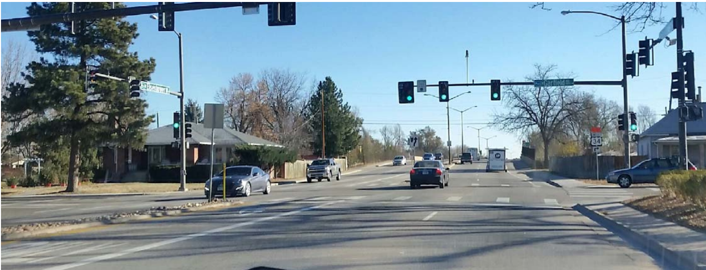
Garfield/US 34 eastbound shows 5 section left turns over left turn lanes, contrary to the current MUTCD.
