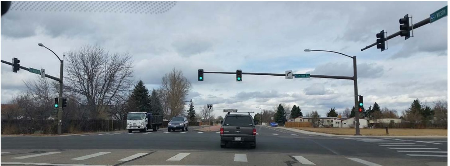
Wilson Ave/14 th Street SW northbound has signal head over left turn and eastbound has no head over left turn lane.
