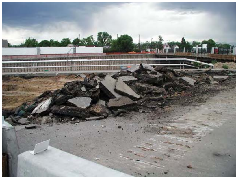
Fig. B1.6.2 Emerson over I-25 – under demolition process
