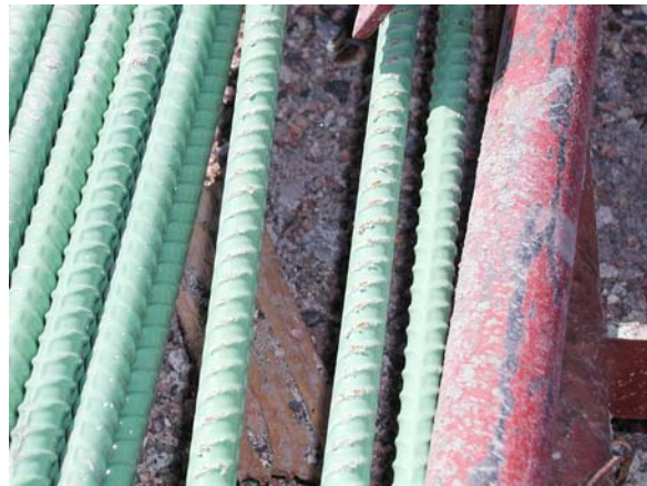
Fig. 2.2 A close view of the epoxy-coated rebars. Surface damages can be seen.
