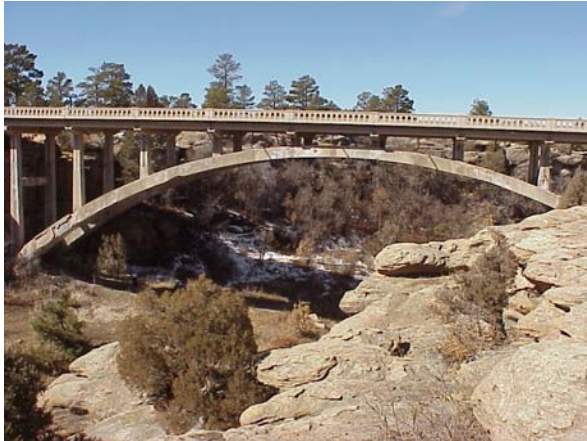
Fig. 3.1 Castlewood Canyon Bridge
