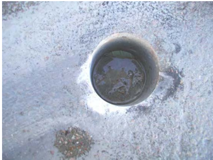
Fig. C.4.9 A core hole in the concrete deck
