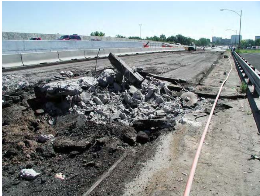
Fig. B1.7.6 Bridge decks under demolition process
