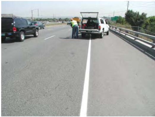
Fig. C.8.4 Cracks on the asphalt overlay (0.013. inch crack)
