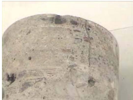
Fig. C.3.13 Cracking in the core
