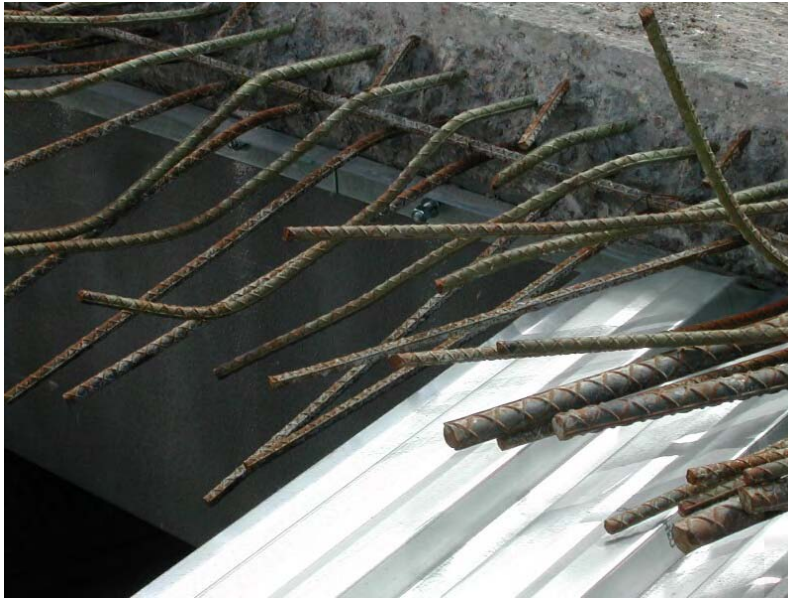
Fig. B1.1.5 A joint between an old and new deck
