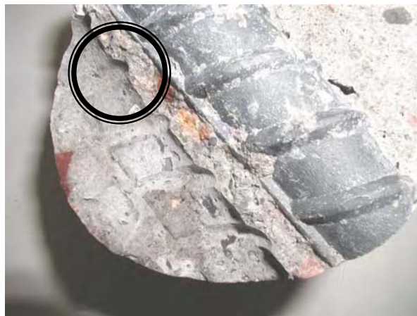
Fig. C.5.12 A close look on the black bar – Rust deposited on the concrete (Concrete with the corrosion inhibitor)
