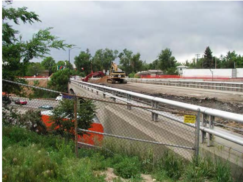
Fig. B1.6.1 Emerson over I-25 – under demolition process
