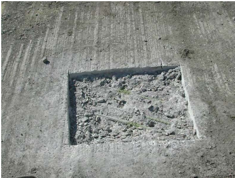
Fig. B1.1.6 Epoxy-coated rebar in a repair patch.
