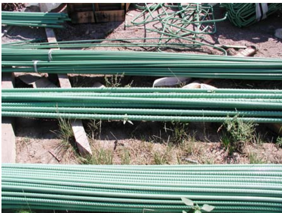
Fig. 2.1 The appearance of epoxy-coated rebars from distance.
