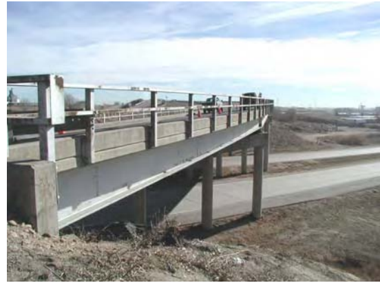
Fig C.1.3 The bridge on the SH 85 in Greeley
