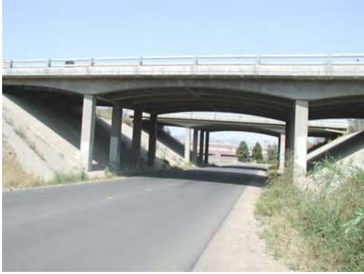
Fig. C.8.2 The side view of the bridge on I70-over Moss St
