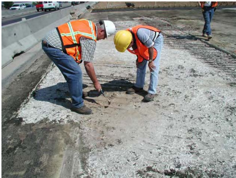
Fig. B1.4.6 Discoloration of concrete deck
