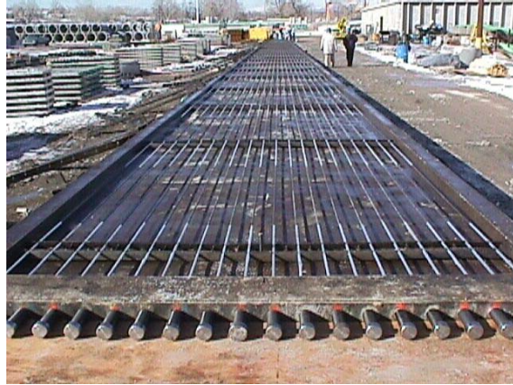
Fig. 3.6 Prestressing bridge decks using CFRP
