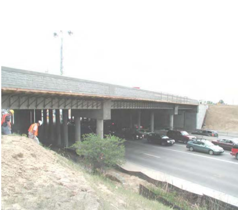
Fig. B1.2.1 Bridge on I-25 over Orchard
