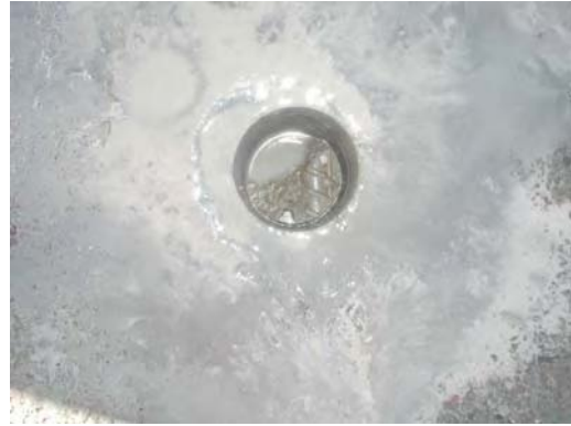
Fig. C.3.9 An epoxy-coated rebar in good condition
