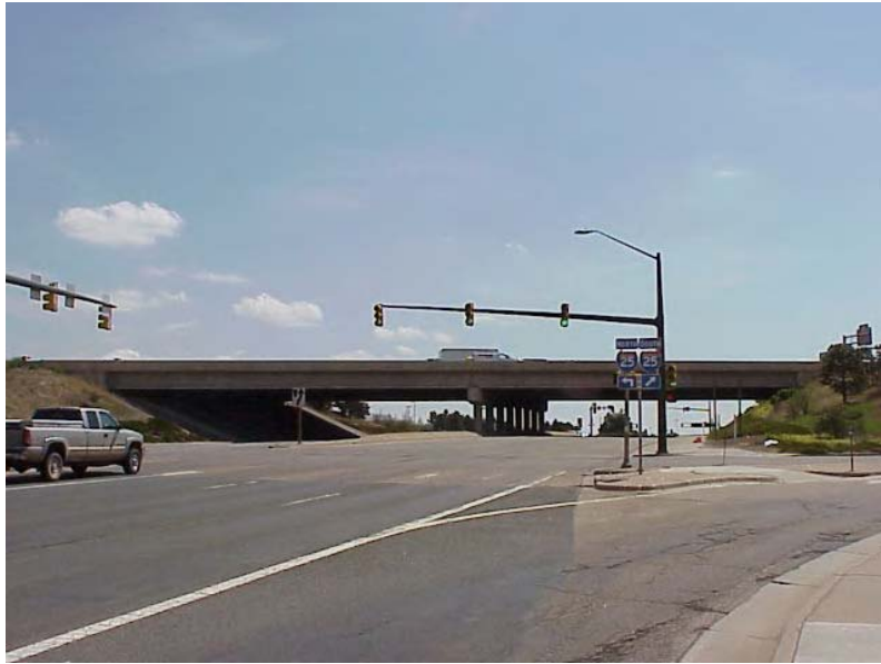
Fig. B1.3.1 Bridge on I-25 over Dry Creek Rd
