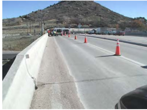
Fig. C.3.3 The bridge surface of Wolfensburger over I 25
