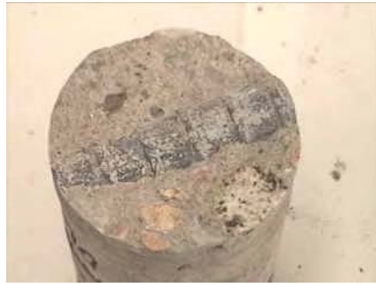
Fig. C.1.13 An extracted steel rebar – in good condition
