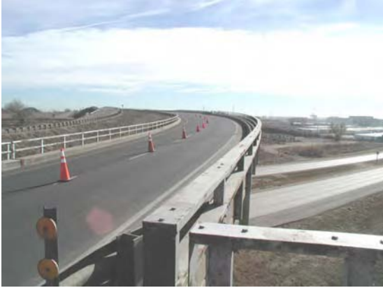
Fig C.1.2 The bridge on SH 85 New asphalt overlay with galvashield corrosion protection
