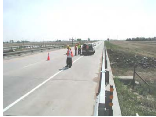
Fig. C.7.3 The bridge surface
