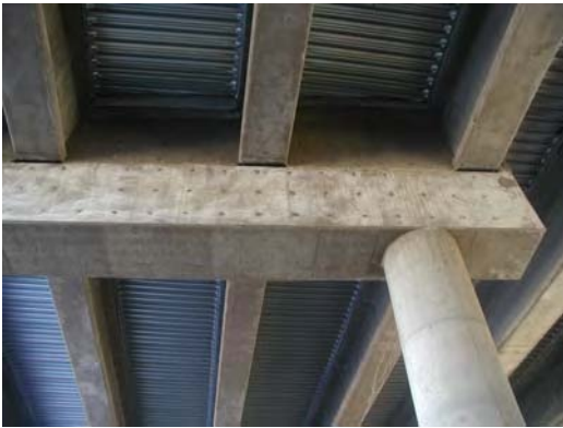
Fig. C.4.4 A bottom view of a pier cap and girder systems
