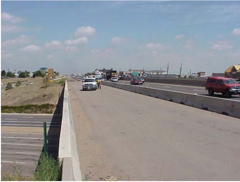
Photo A.3.3 Bridge deck – asphalt overlay
