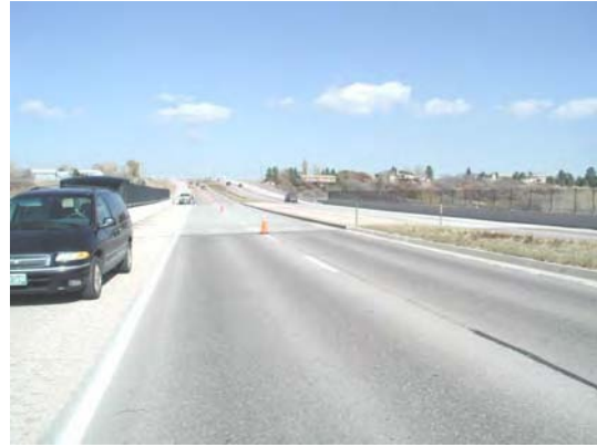
Fig. C.5.3 The bridge surface on SH 83 in Colorado Springs
