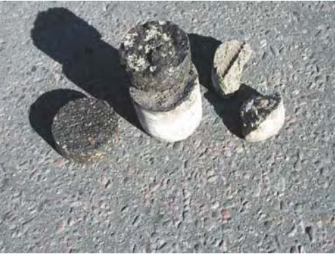
Fig. C.9.6 Concrete cores extracted from the driving lane
