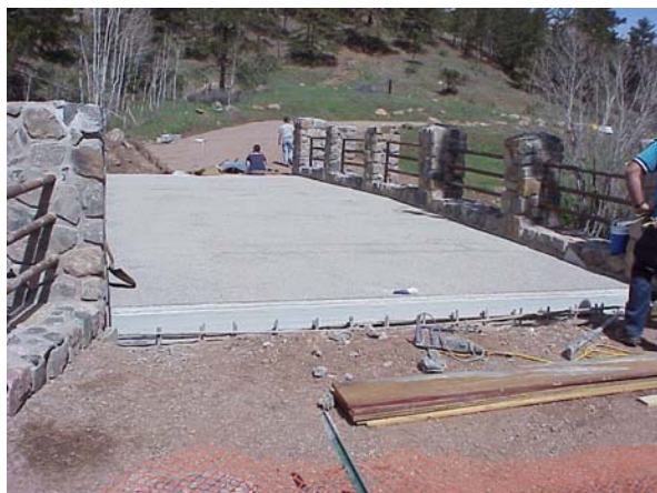
Fig. 3.7 Installation of GFRP decks in O’Fallon Park Bridge (Denver, Colorado).
