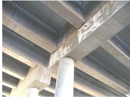
Fig. C.4.5 A bottom view of a pier cap and girder systems
