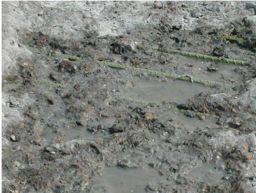
Fig. B1.1.4 Epoxy-coated rebars – in good condition
