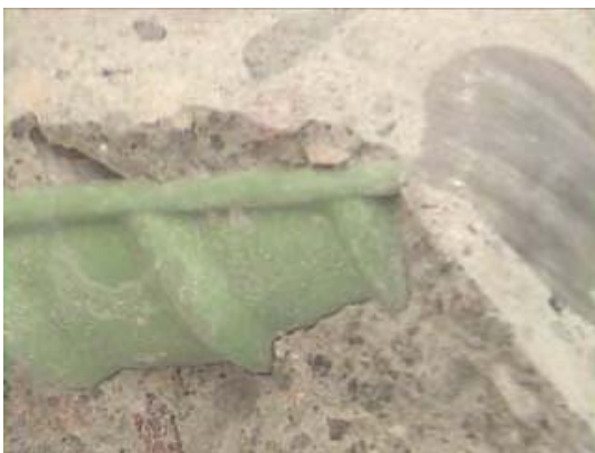
Fig. C.3.12 A close look on the epoxy-coated steel rebar – in good condition
