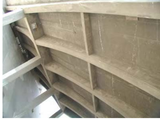
Fig. C.8.3 The bottom view of the girder system
