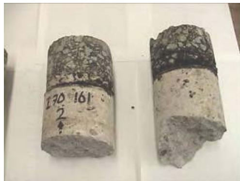
Fig. C.8.12 Concrete cores taken from the driving lane
