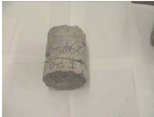
Fig. C.7.10 The delamination in the concrete overlay
