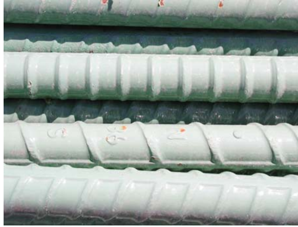
Fig. 2.3 A close view of the epoxy-coated rebars. Corrosion started on the locations with damaged coatings.
