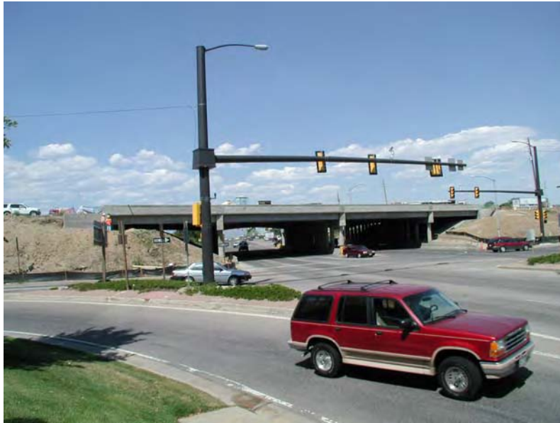
Fig. B1.4.1 Bridge on I-25 over North Bound Belleview
