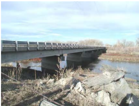
Fig. C.2.2 The bridge on SH 34 Business Route
