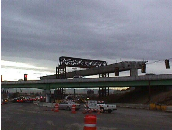
Fig. 3.5 I-225 & Parker Interchange project
