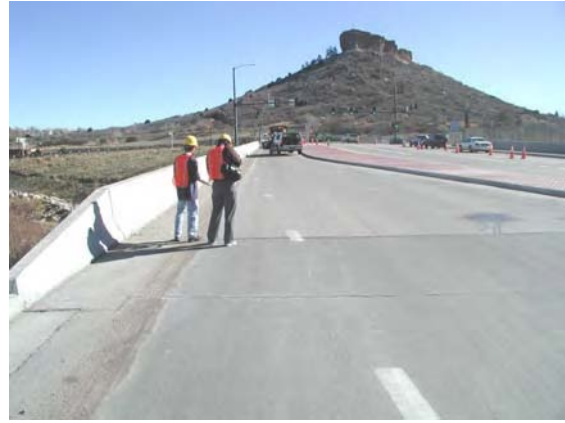
Fig. C.4.3 The bridge surface of Wolfensburger Road WB over Plum Creek
