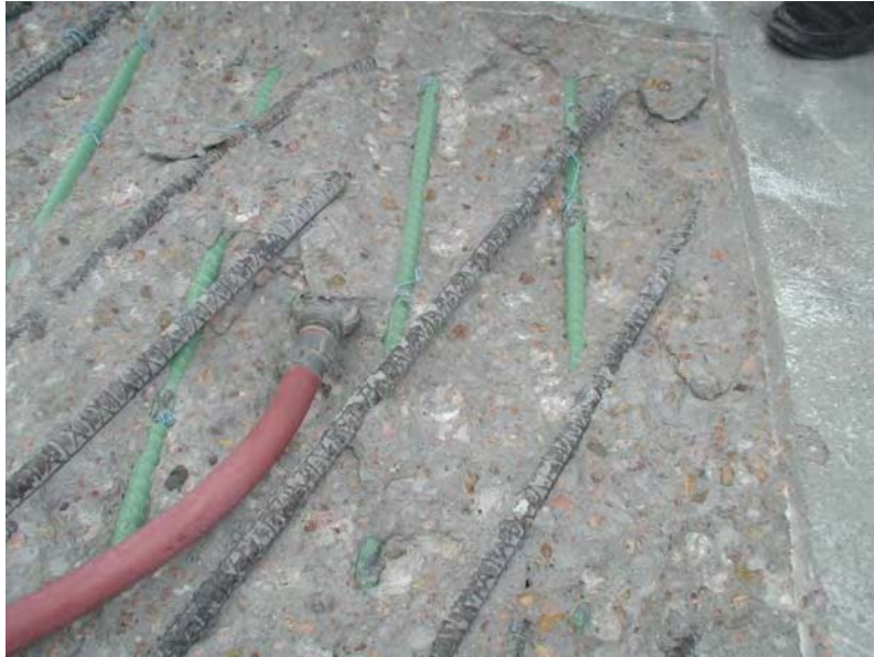
Fig. B1.2.5 Some black bars (1970's part) are in good condition.
